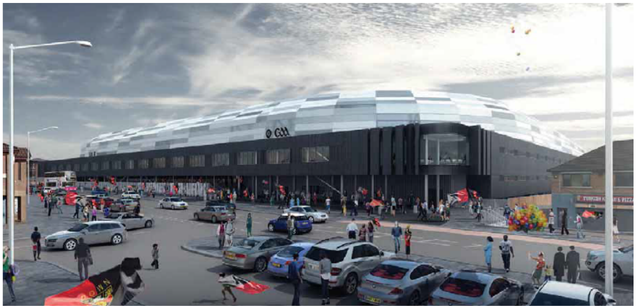
Andersonstown Road Facade looking east
